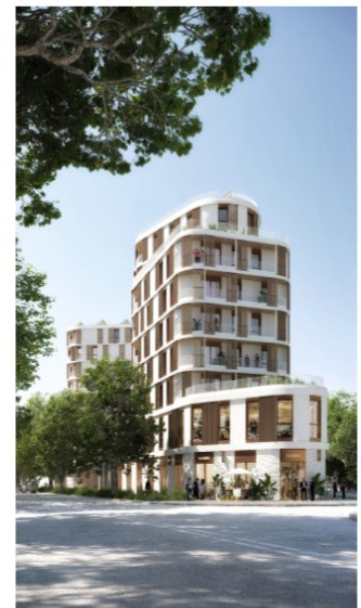
FLORA PARIS, FR (IN CONSTRUCTION)
